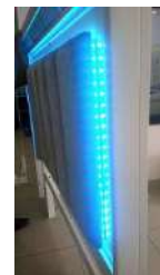
LED lighting (Blue)
